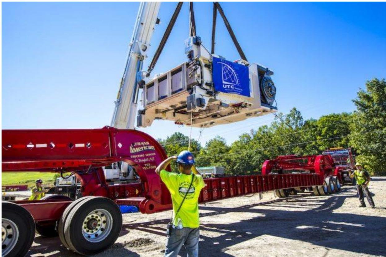
Gently does it: a 60t cupping press is lifted off an eight-axle trailer
