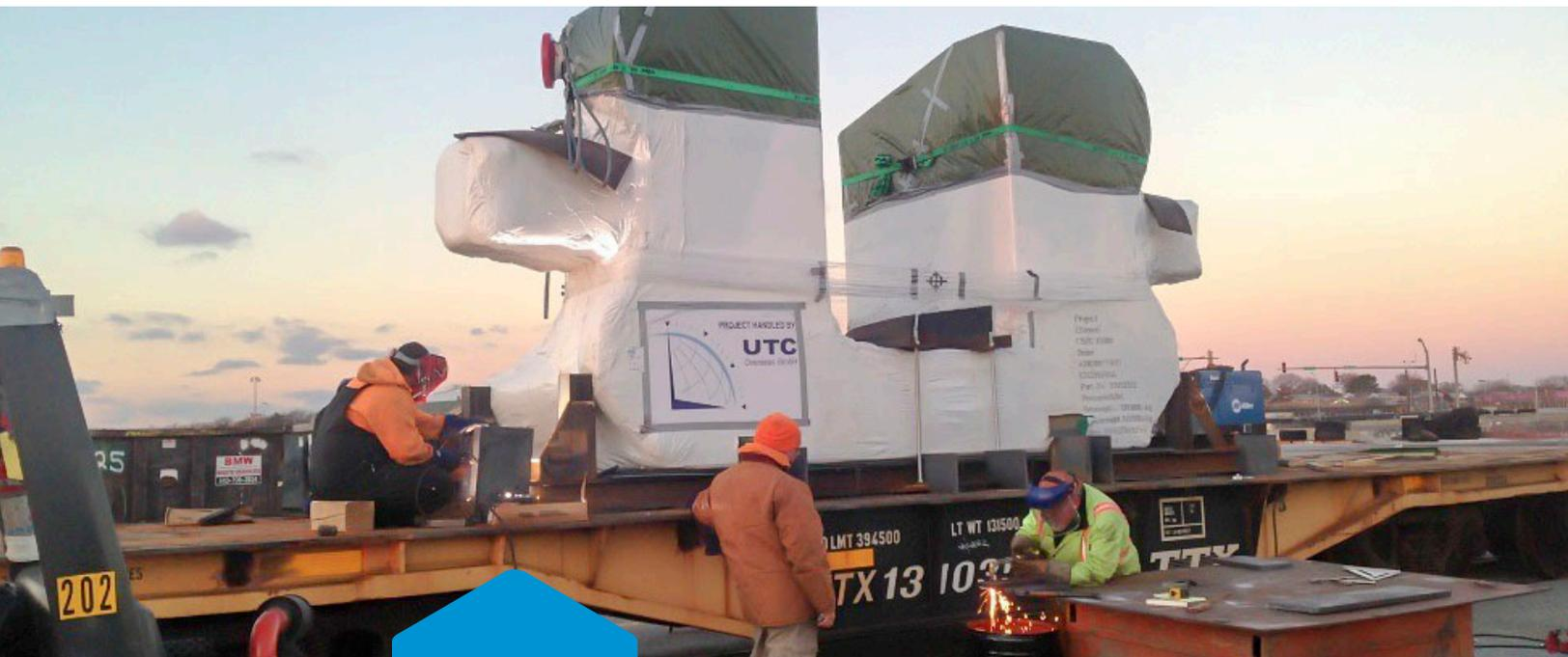
Riggers secure heavy components of the press to railcars at the Port of Baltimore for transport to the Pennsylvania jobsite. In all, 221 forge pieces, with a combined weight of over 1,870 tons/1699 MT were transported.
